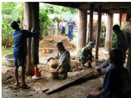
The lifting of an old wooden house to add new concrete foundations beneath existing columns to preserve the house (2011).
